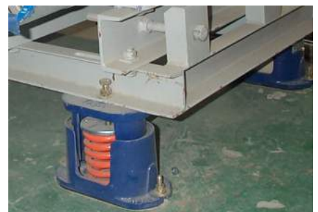
VENTILATION UNIT DETAIL
